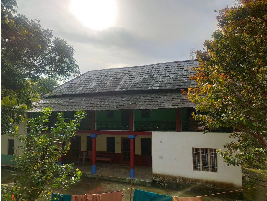
Figure 1: A typical vernacular house in the study area
