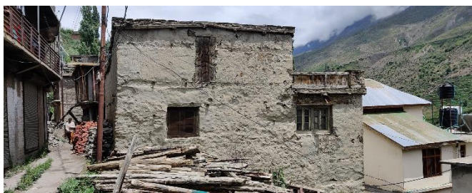
Figure 17. Outer Building wall facade (Source - Author)
