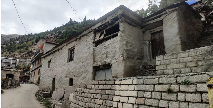
Figure 2. Vernacular Architecture of Keylong Region (Source: Author)
