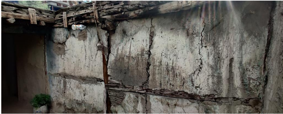
Figure 20. Wattle and daub detail (Source - Author)
