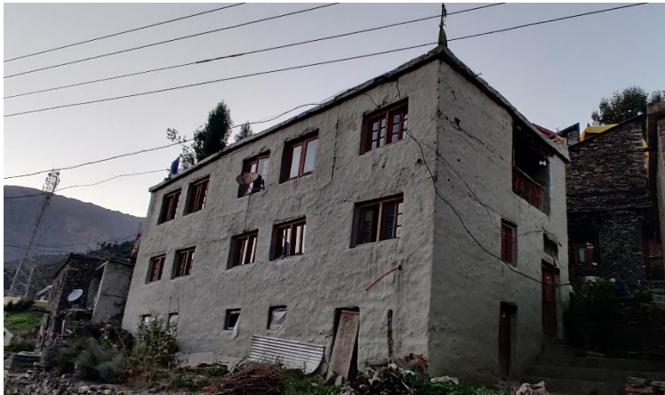
Figure 1. Vernacular architecture of Keylong Region (Source: Author)
