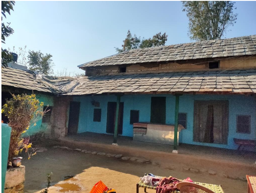
Figure 3: A typical vernacular house in the study area
