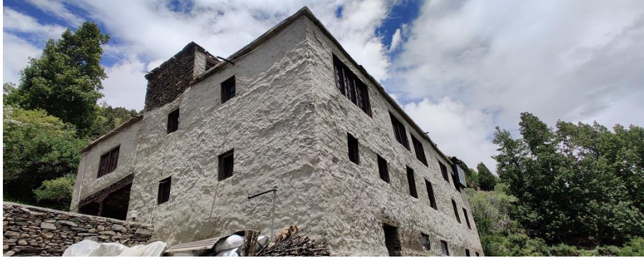
Figure 26. Building openings (Source - Author)
