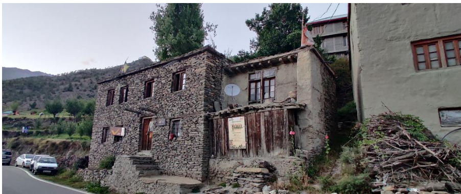
Figure 8. Local Vernacular Architecture Example (Source - Author)
