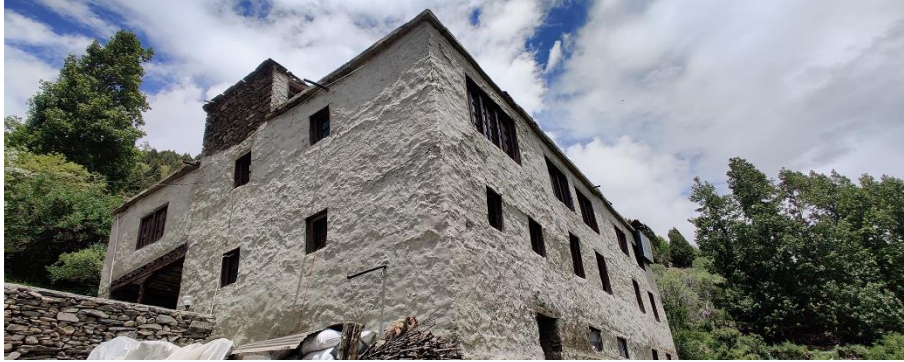
Figure 26. Building openings (Source - Author)
