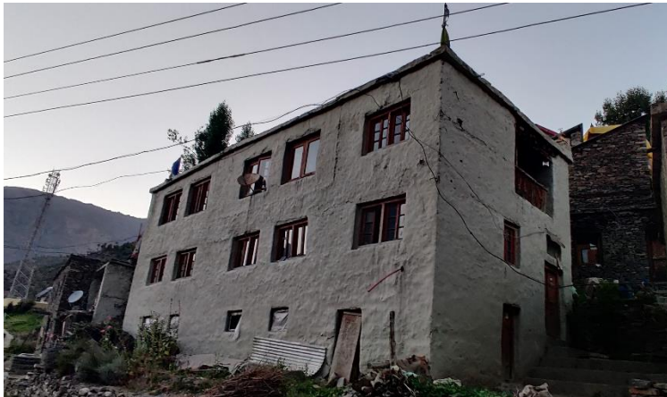
Figure 1. Vernacular architecture of Keylong Region (Source: Author)
