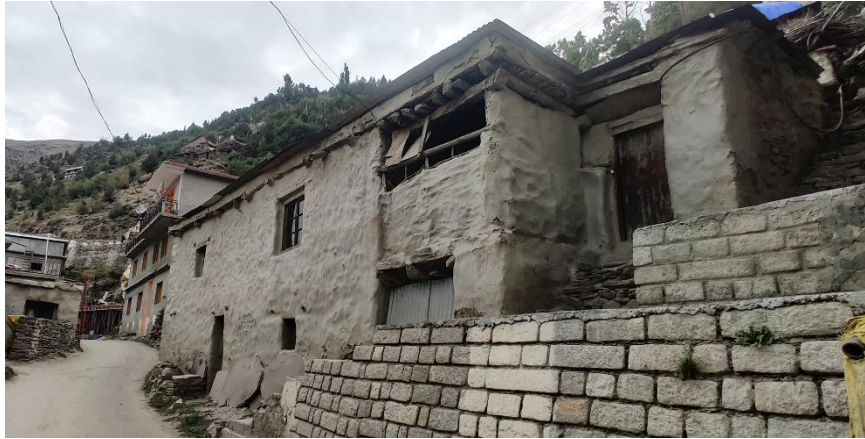
Figure 2. Vernacular Architecture of Keylong Region (Source: Author)
