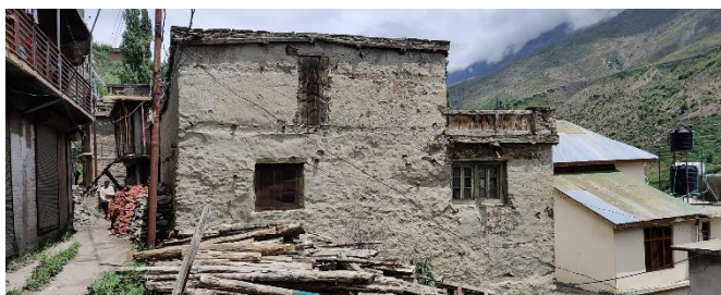
Figure 17. Outer Building wall facade (Source - Author)
