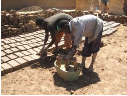
Fig. 3 - Manual brick forming.
