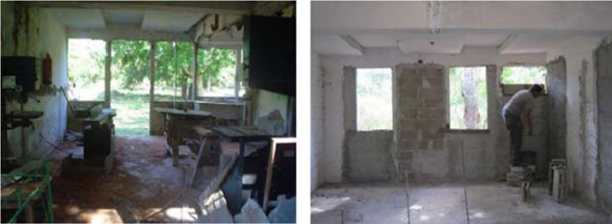
Fig. 12, 13 - Project “Habana-Ecopolis” – Marianao (internal restructuring).
