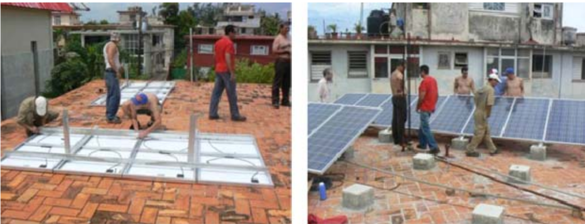
Fig. 14, 15 - Project “Habana-Ecopolis” – Marianao (installing solar panels).
