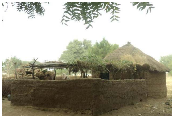
Fig. 2 - House in crude earthen bricks in the Logone valley.
