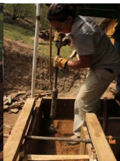
Fig. 11 - Compaction with pneumatic piston.
