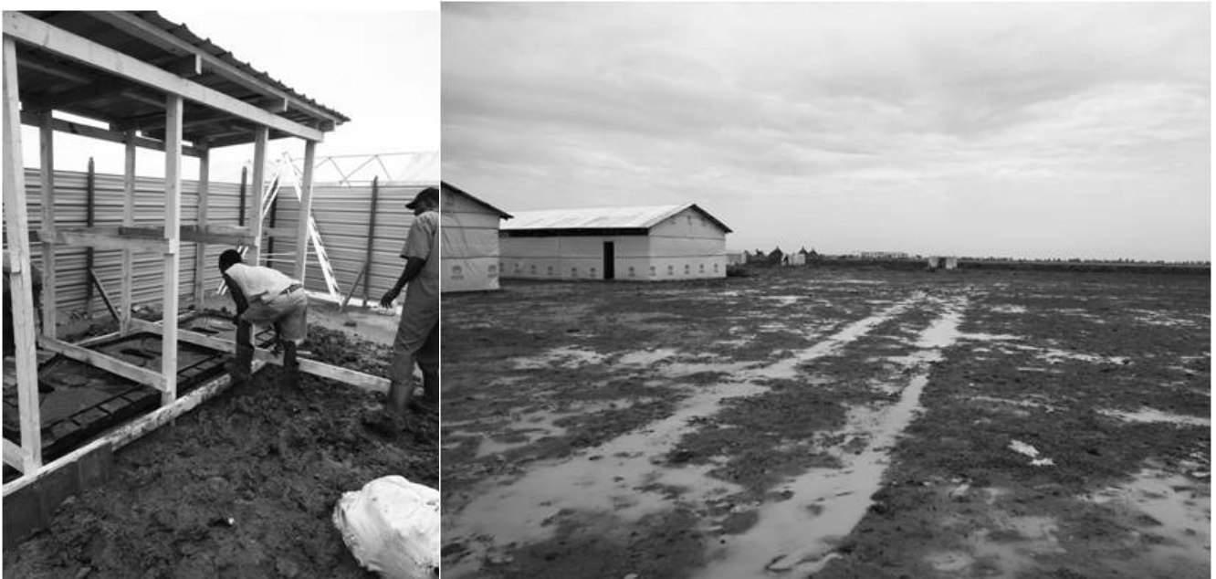
Fig. 4 - Latrine Construction, Nyeel Refugee Camp, South Sudan ( source: FAREstudio_2013 ).
