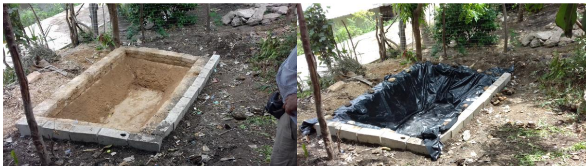
Figure 4 – New cistern prototype. Left: no plastic coating, right, with coating (Photos: May 2017).
