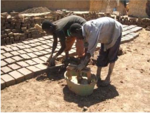
**Fig. 3** - Manual brick forming.
